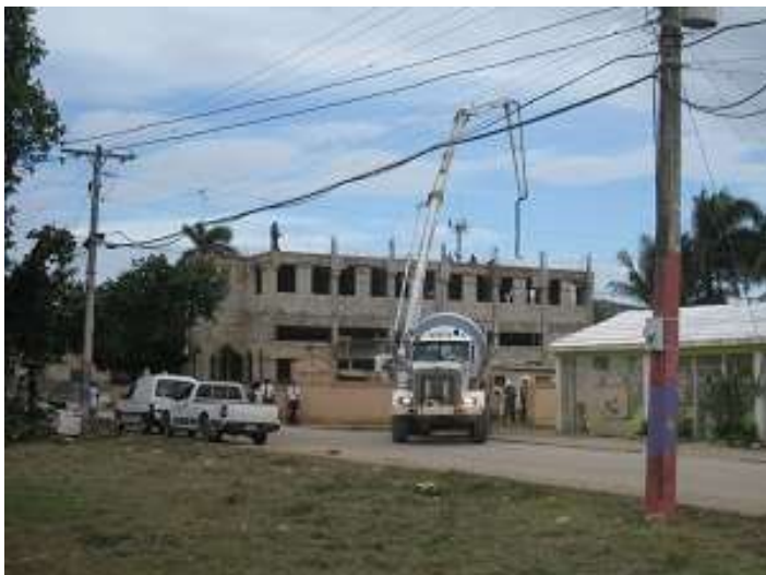
The roof is being poured, summer 2013.
