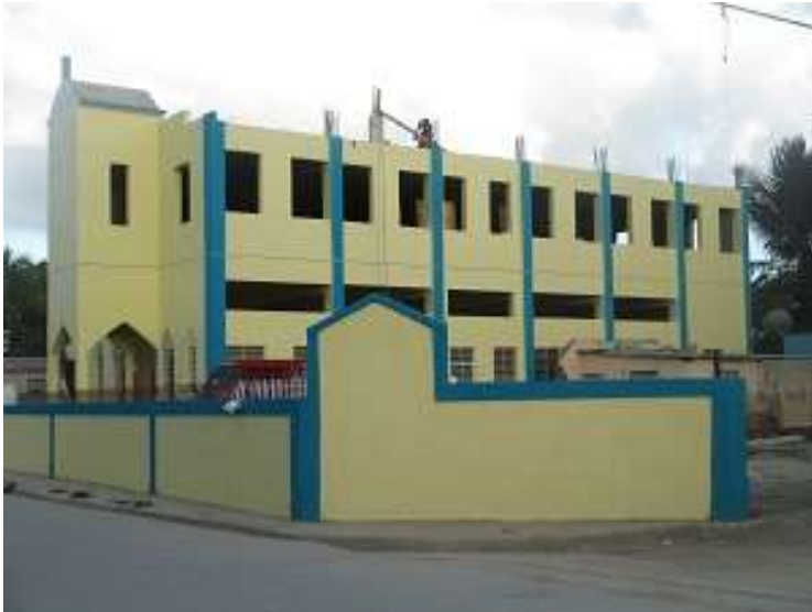
Outside view after teams were done at the end of June 2014.
